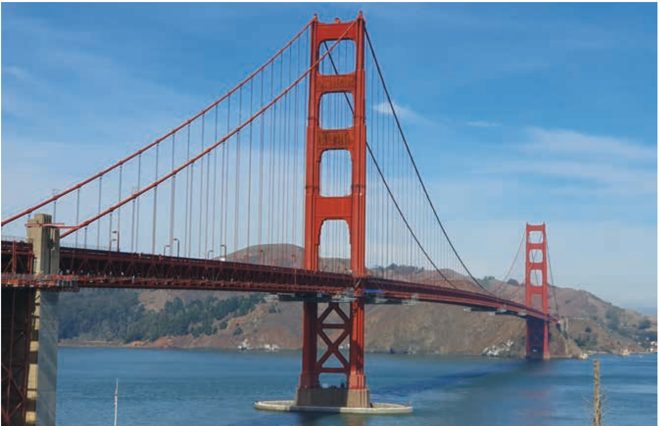
Golden Gate Bridge
